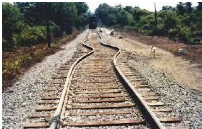
Railways deformation caused by extreme heat in Europe in 2023
